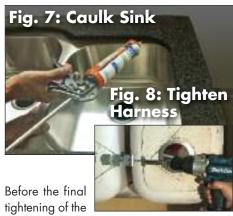
Sink Harness, run a bead of silicone caulk around the undermount sink lip to create a watertight seal. Tip: With a (cordless) drill, It's fast and easy to tighten the Harness underneath an installed sink. As it tightens, the Harness will lift the sink up into position and hold it there. When properly installed, the Universal Sink Harness will withstand up to 200-250 lbs.of load.
