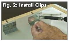
Insert supplied wire up through a clip hole and bend into a "V" shape. Bend the upper end underneath lower end to make a bend in the wire, then bring over into a knot, and crimp the wire to set it with pliers. Repeat steps to attach the lose end of wire into the second clip to make a "V". The end of the "V" shaped wire should be 2-3 inches from the center of the sink installation area.
